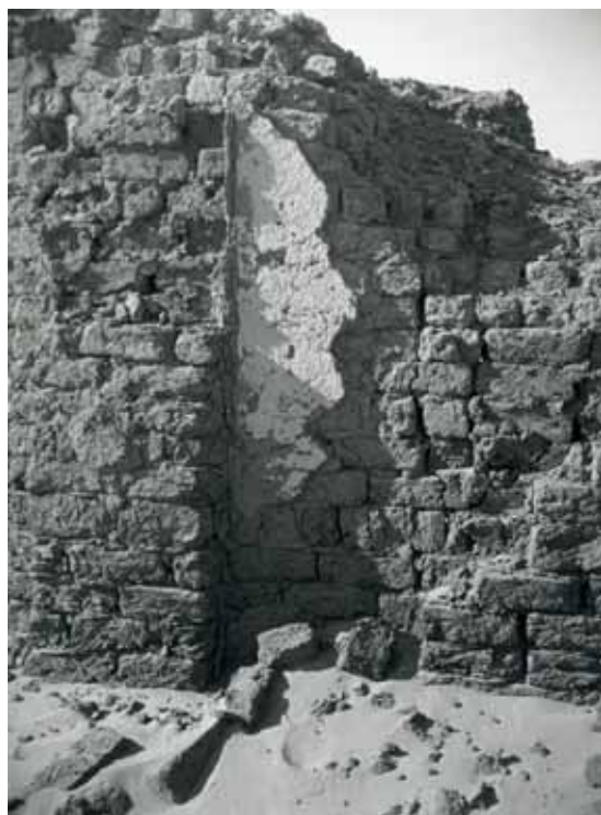
Fig. 54. Abydos: Shunet es Zebib [storehouse of raisins], ancient wall covering of mud plaster
