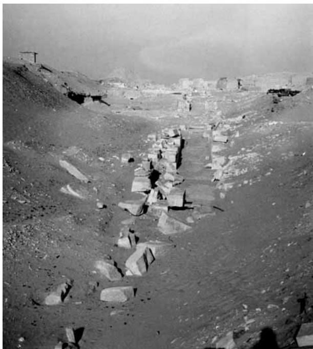
Fig. 69. Saqqara: Unas Causeway, looking west, towards bend
