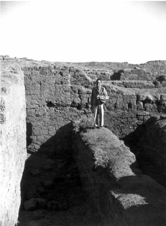
Fig. 51. Deir el Ballas: North Palace, interior with François Daumas (1915–1984)
